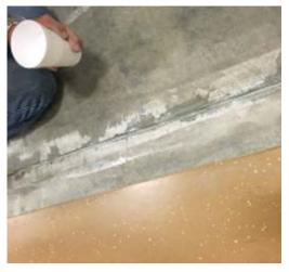
3) After mixing 670 to flowing consistency, use a mortar bag to dispense into cracks
