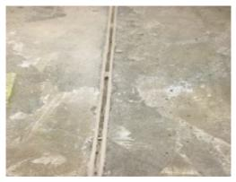
2) Using a small paint brush apply a coating of the 670 Acrylic primer along the walls and bottom of joints
